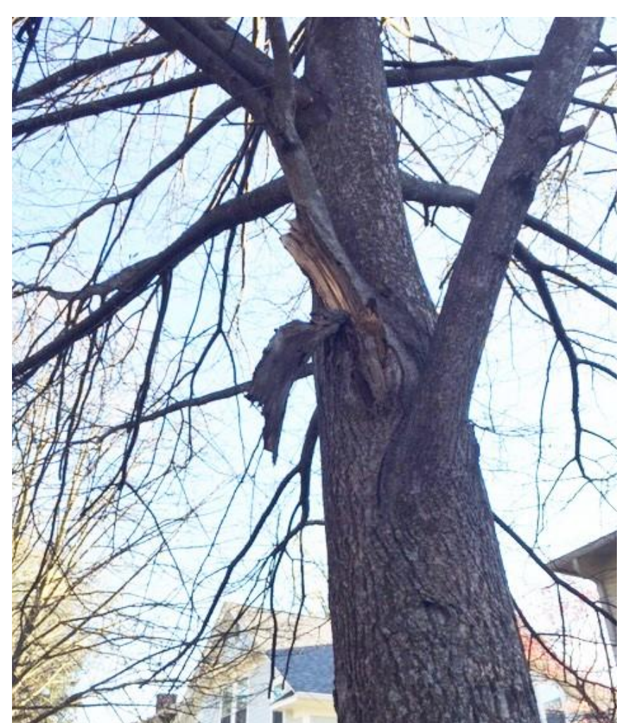
Figure 2. Tree requiring maintenance
