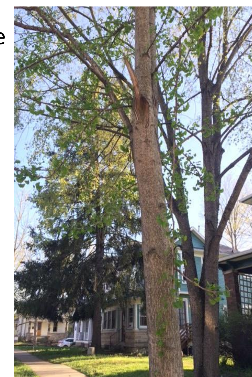
Figure 5. Tree requiring maintenance
